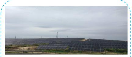
In late June 2016, we connected a 50 MW "Top Runner" project in Datong City, Shanxi Province to the grid. The project utilized Yingli's TwinMAX 60 Cell bifacial series module, a frameless dual glass module that integrates Yingli's cutting-edge PANDA (n-type monocrystalline solar cell) technology which leads to a module efficiency of up to 18.8%.
